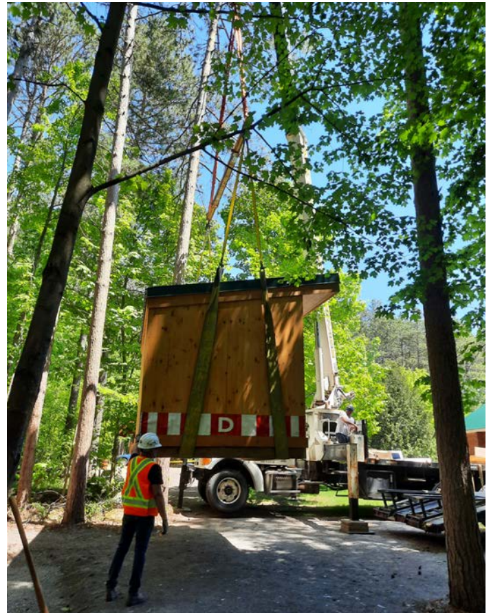
Crane lowering red pine CLT HUTT into place at Limerick Forest.
